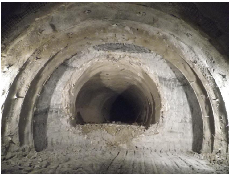
View of the NATM tunnel with the exploratory tunnel
