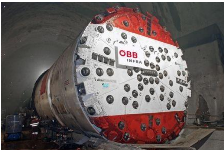
TBM in assembling chamber South(KAT2)
