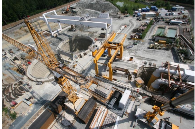
View of the site installation area of the Koralm tunnel KAT2
